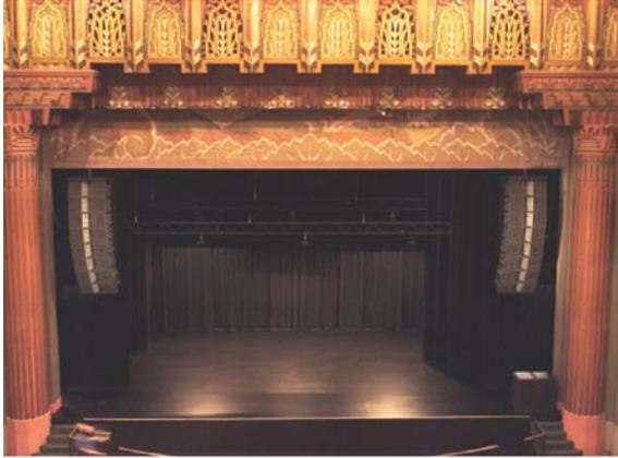
Figure #9. : Left/Right VT4889 Arrays in Proscenium Stage Theater (pair of 8-box arrays)
