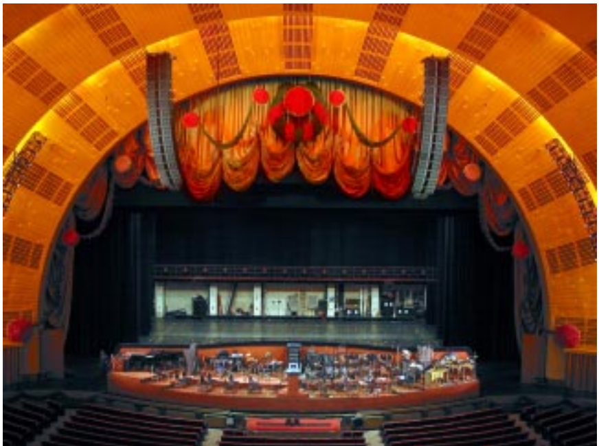
The Great Stage at Radio City Music Hall for the Radio City Christmas Spectacular. The Sound System includes two arrays of VERTEC line array speakers from JBL powered by Crown amplifiers.
