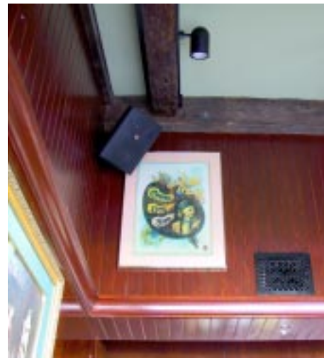
Detailed view of Control 25AV in place
