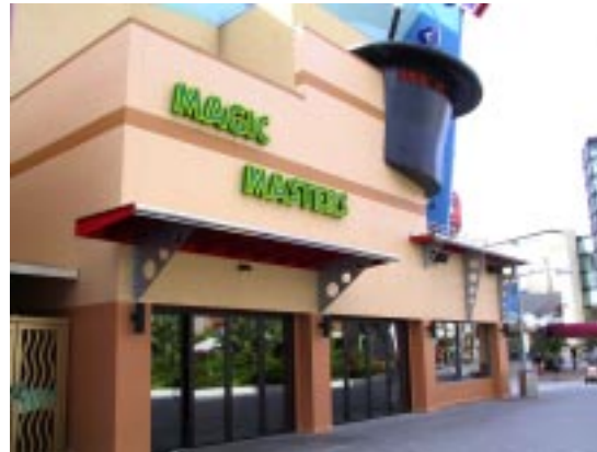
Magic Masters in Downtown Disney: JBL Control 29AV visible under rear awning
