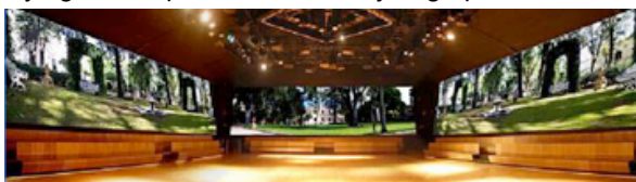
Vitel S.A. recently installed an immersive JBL loudspeaker system at the “Jerez’s Mystery” exhibit at the Atalaya Museum in Spain.
