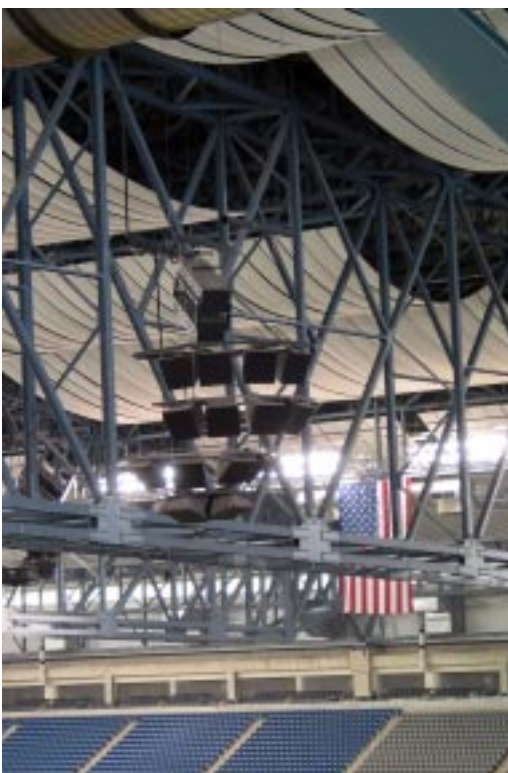
One of four endzone arrays of PD Series Loudspeakers at Ford Field, Detroit.
