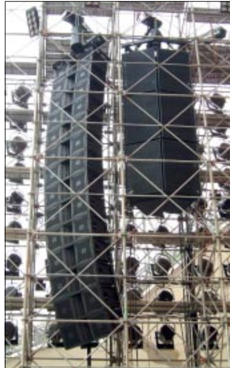
One of two speaker and lighting towers on either side of the stage at Hong Kou stadium. Fourteen VERTEC VT4889 Line Array speakers and six HLA 4895 speakers are on each tower.
