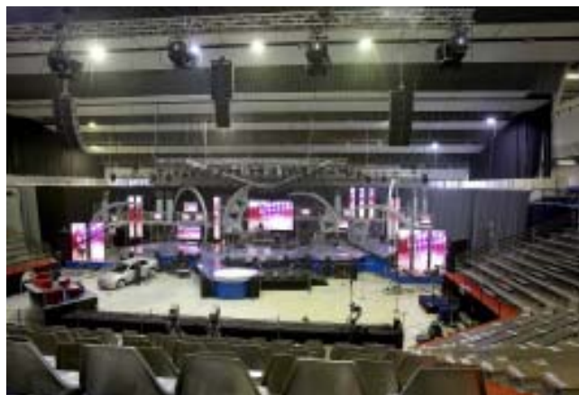
Amex Audio provided a JBL VERTEC line array system for Superstar 2006, one of Slovakia's most popular live televised shows. VT4889 full size and VT4887 compact models were used to address the challenging architectural features of Bratislava's Incheba Hall C.
